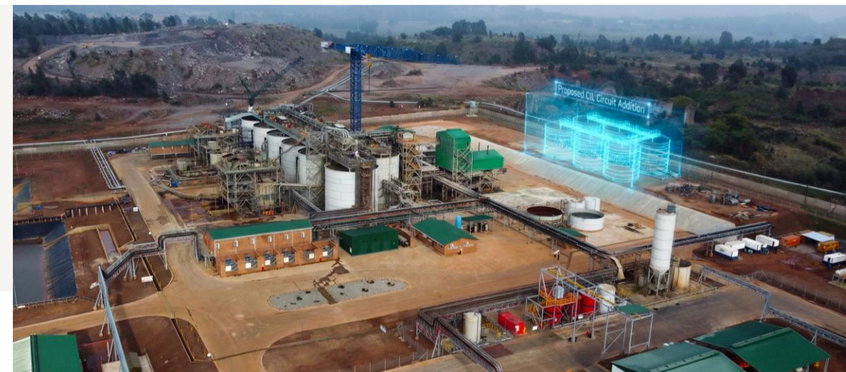
Proposed STR circuit CIL tanks at MTR
