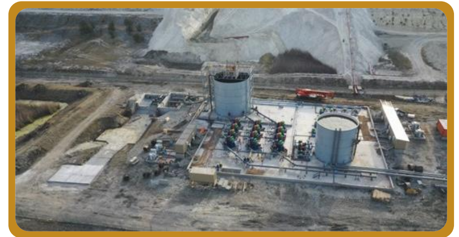
Leslie/Bracken pump station under construction at Elikhulu
