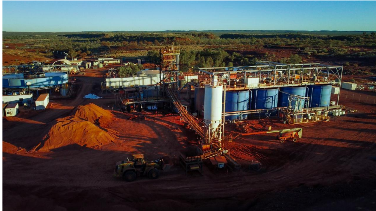
TCMG Nobles Gold processing plant
