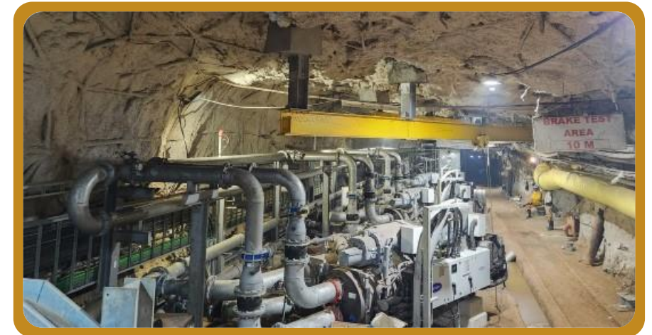
Phase 1 of underground refrigeration plant at Evander 24 Level
