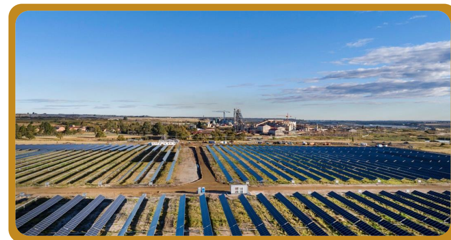
Solar PV plant at Evander Gold Mine
