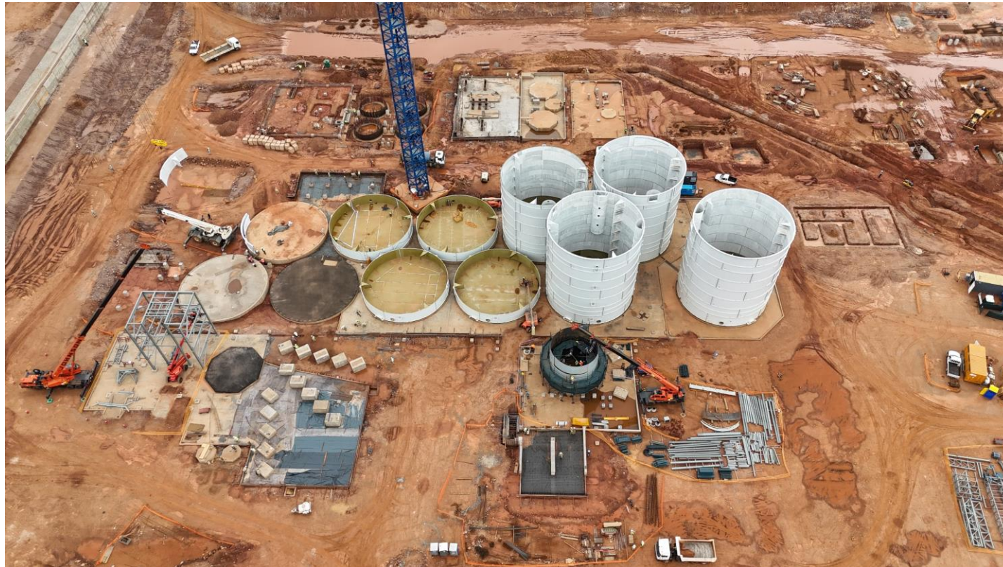
MTR processing plant under construction
