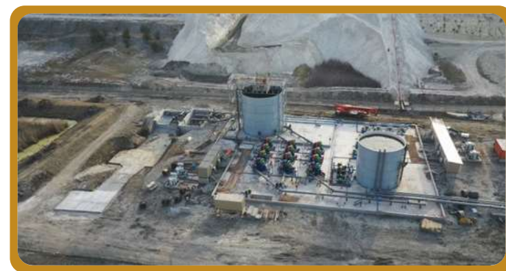
Leslie/Bracken pump station under construction at Elikhulu
