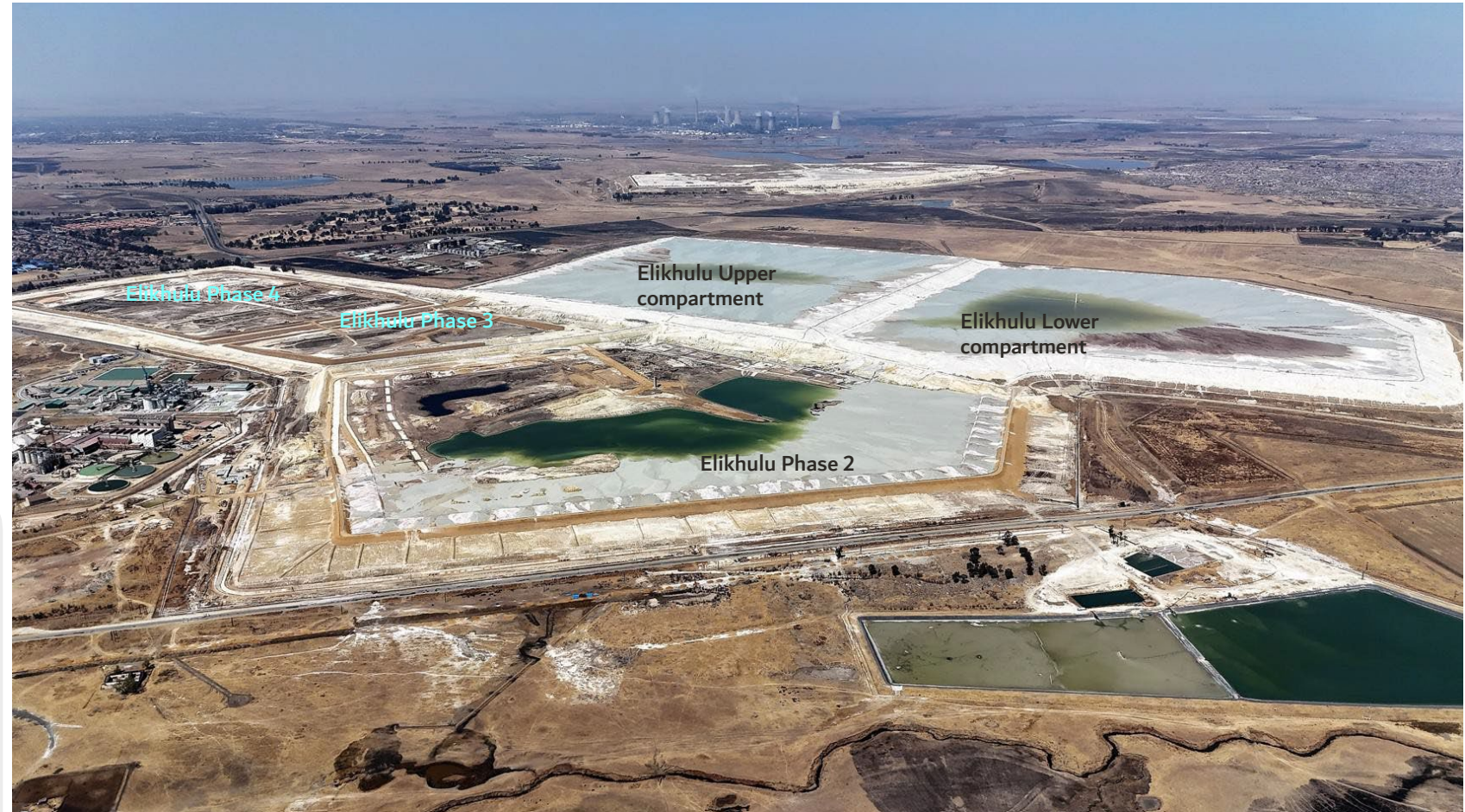
Elikhulu TSF Complex
