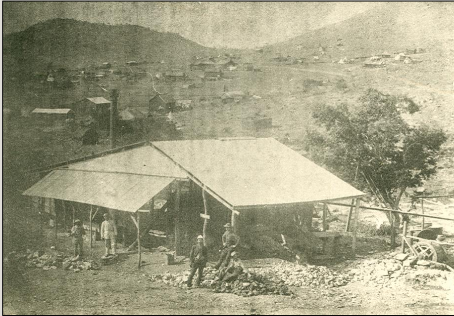
The central mill at Barberton, near Rimer's Creek. The small workings could bring there ore here to be toll treated.
