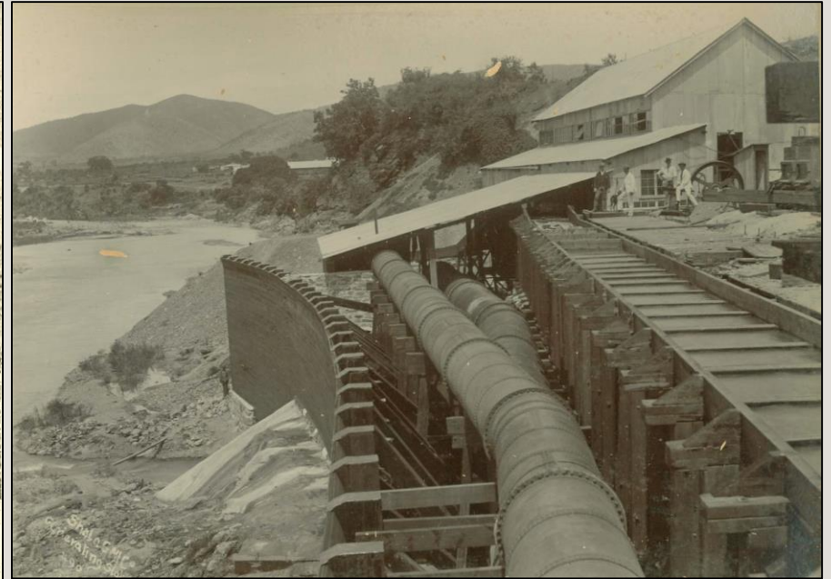
06-463-41 Sheba GMCo generating station
