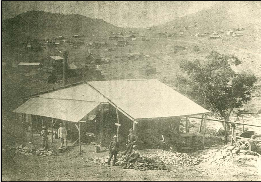
The central mill at Barberton, near Rimer's Creek. The small workings could bring their ore here to be toll treated.
