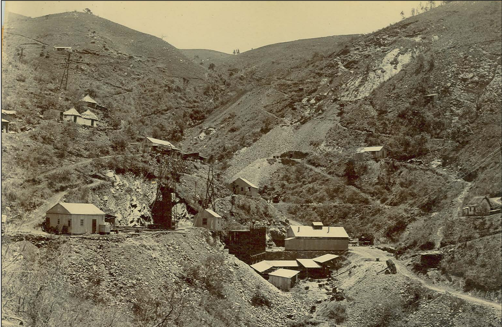
Sheba mine, with the Soper shaft in the foreground
