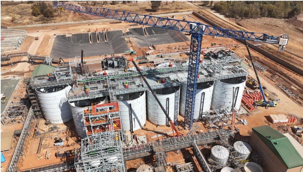
MTR processing plant - Construction nearing completion
