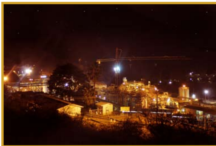
BIOX® Plant - Fairview
